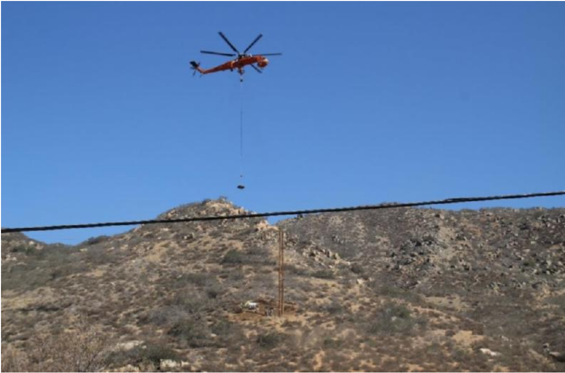
Photo depicting helicopter placement of the approximately 7,000 lb. micropile cap plate
