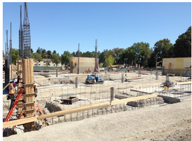
Garage Foundation under Construction
