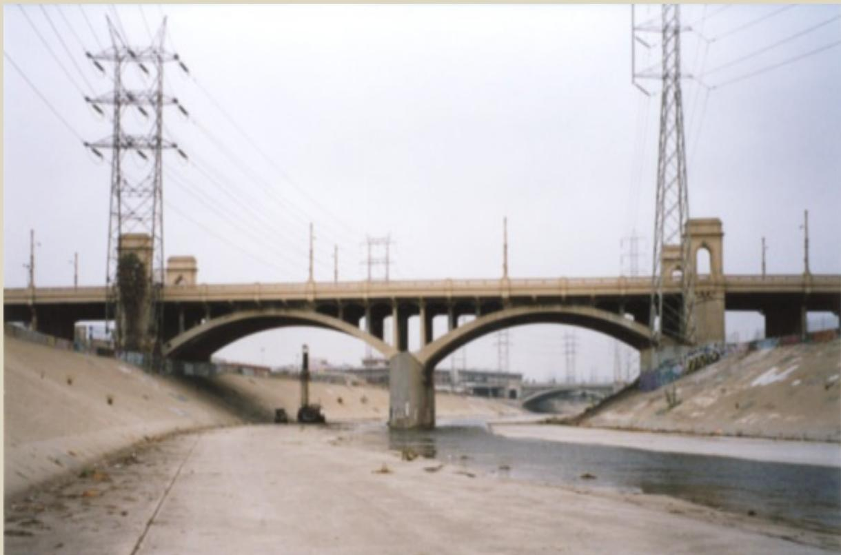
The riverbed geology included loose, liquefiable sandy soils with many dense gravel bars, cobble and boulder pockets to 50 feet, dense sands to 70 feet and Siltstone bedrock below. The bridge has 29 bents and
