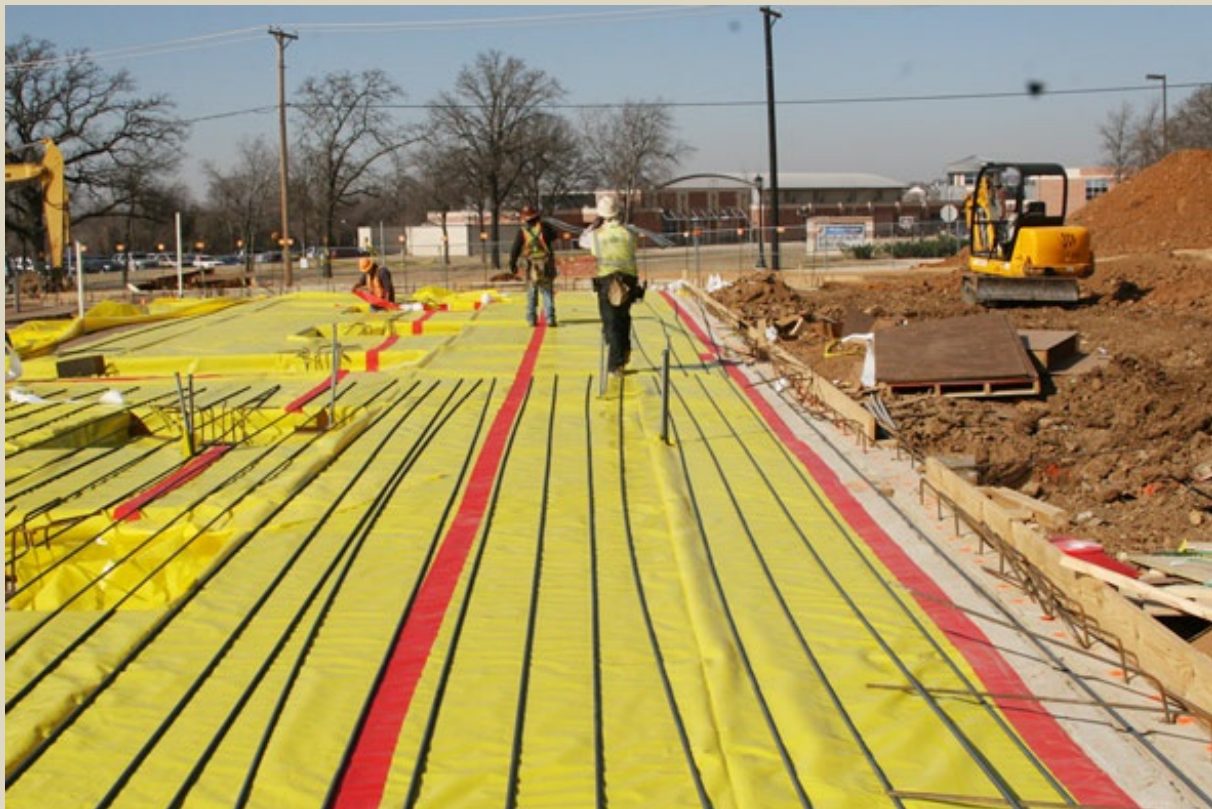
Crete Claw Installation
