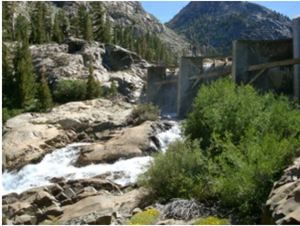
View from the Agnew Lake Dam spillway
