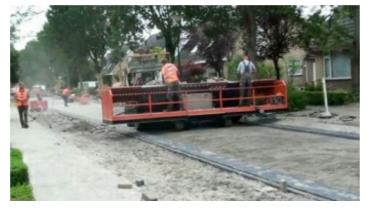
We don't have many brick-paved public roads in California, but apparently they have enough in Holland to warrant developing a brick laying paving machine. Tiger-Stone is a Dutch paver laying machine that produces brick roads. Paving bricks are dropped into the angled trough by a front-end-loader. Men help to spread them in the trough as they drop into the forming jig. As the electrically operated crawler moves forward along a pre-laid sand base layer, all the bricks are packed, held
