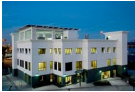
Port of Long Beach Security Command and Control Center
